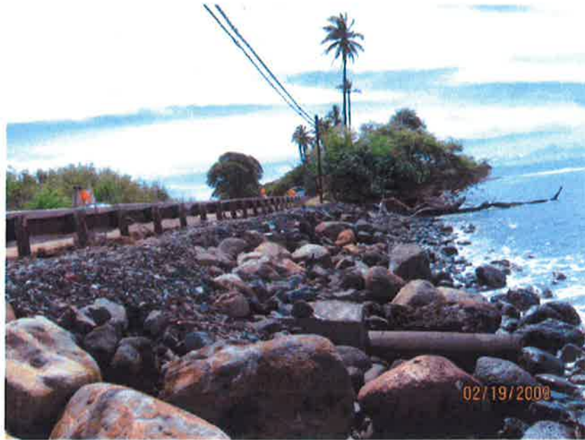
Photo No. 1. View of Shoreline Facing South
